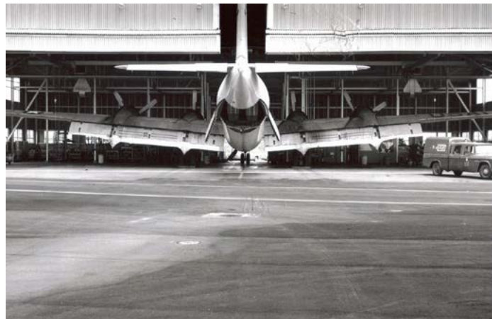
A Delaware Air National Guard C-97 Stratofreighter receives maintenance in the old fuel cell, circa mid 1960s. This original fuel cell hangar was constructed in 1962 and is scheduled to be demolished and replaced. (Photo courtesy of the Delaware Military Museum)
